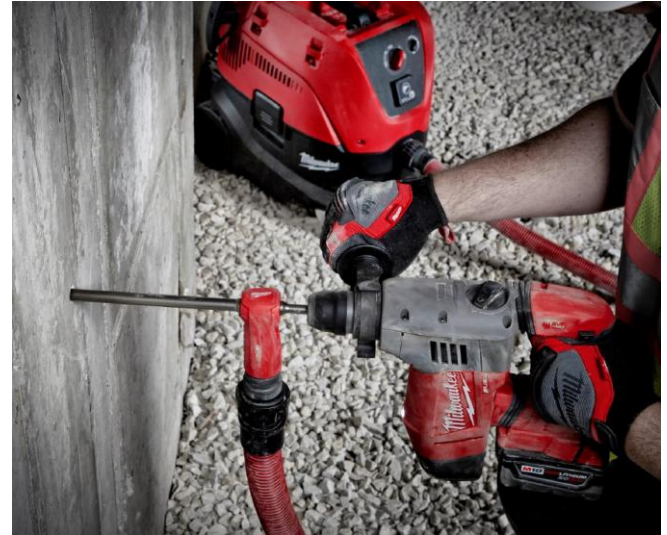
Hollow Vacuum Drill Hole Preparation
